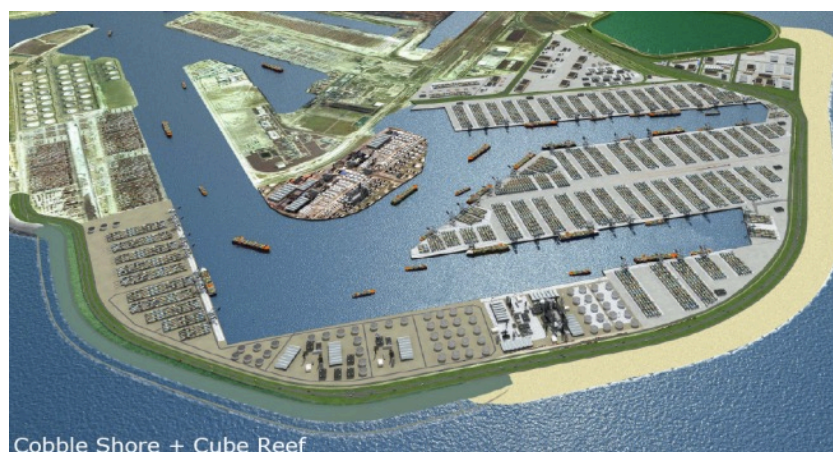
Figure 4: Maasvlakte 2 with hard sea defense design and built (Loman, 2012)
