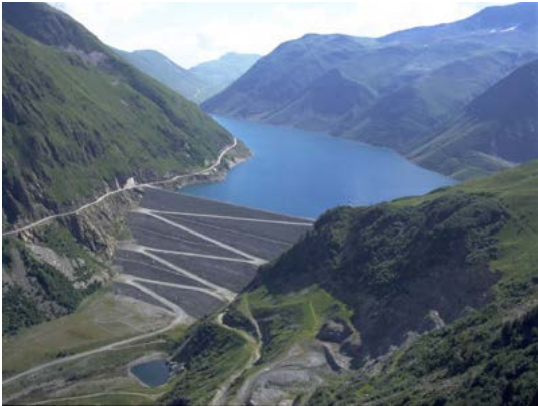
Figure A.11: View of the dam and reservoir of the Grand'Maison Storage Pump Station.
