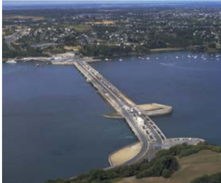
Figure A.2: La Rance Tidal Power Station. source: https://tethys.pnnl.gov/annex-iv-sites/la-rance-tidal-barrage
