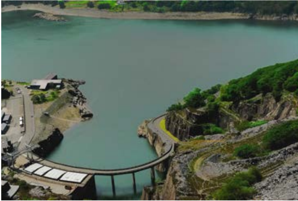
Figure A.12: View of the reservoir of the Dinorwig Storage Pump Station.
