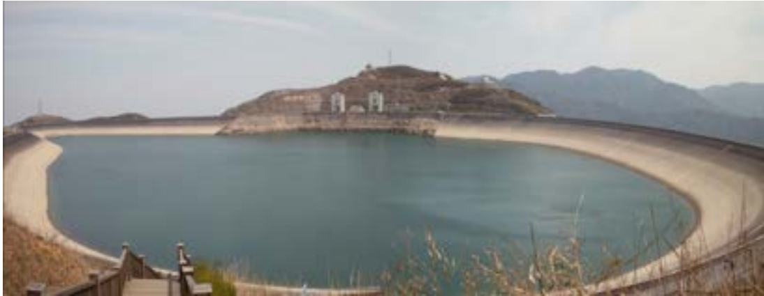
Figure A.10: Tianhuangping Pumped Storage Station
